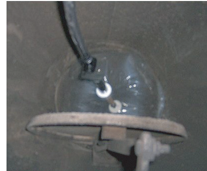
Chimney Balloon Installed
